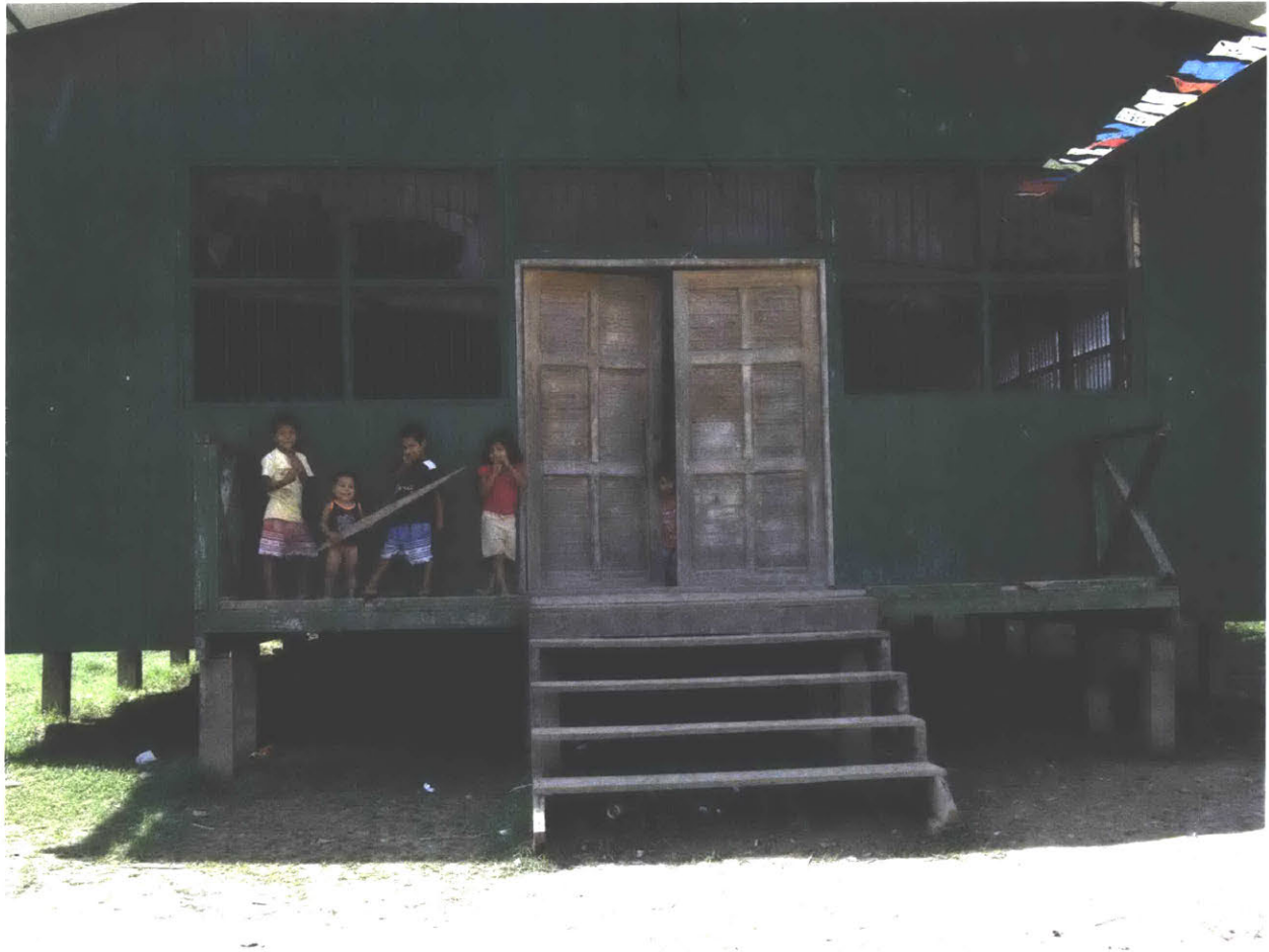
The community hall in Paoyhan is built on stilts, for when the floods come. Photo by Laura Dev.
