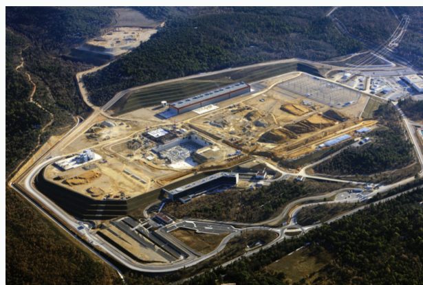
The construction site of ITER in southern France. Image: ITER.
