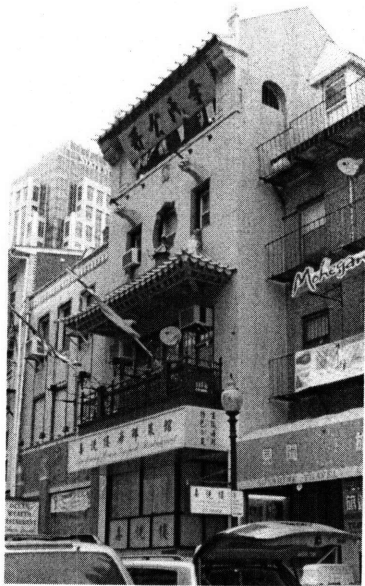
Figure 1-28. The Goon Shee-Lee Association Building at 10 Tyler Street.
